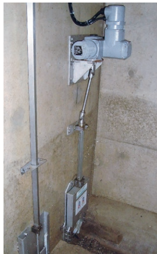
EasySlide actuator and special slide valve with connection to a central control
